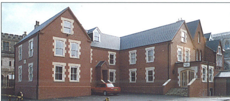
Client: Ringrose & Co. Solicitors, Boston. Contractor: H. H. Adkins (Contractors) Ltd., Boston.
