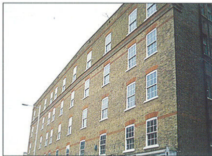
Client: Alan Selby & Partners. Contractor: Halstead Contracts Ltd.
